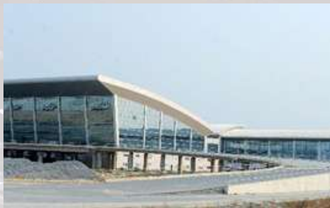
Figure 9 – Works on the New Luanda International Airport
